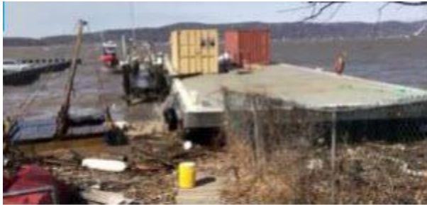
The runaway barge (seen here alongside Irvington Boat Club's pier) smashed into and damaged the pier during a storm on May 2, 2018. Photo: Irvington Boat Club
